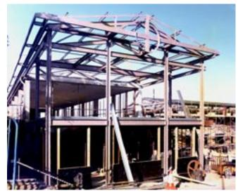
BEFORE: The Concrete frame of the Gatehouse was extended in steel. Steel is like the whalebone in corsetry. Why use anything so easily rusted, and melted, and so conducive of noise and heat, for anything except its enormous strength and stiffness?
