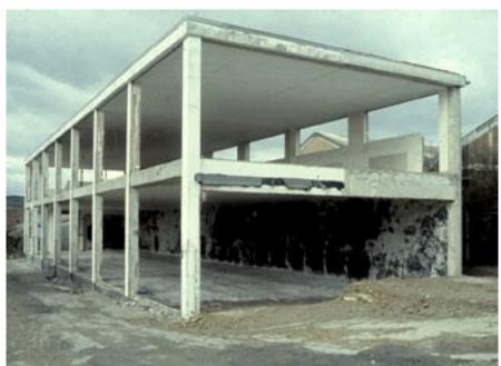
BEFORE: The 'Gatehouse Block', stripped down to its frame and floors. This almost completely useless object was published by Corbusier as the 'Essence of Architecture'. Neither he, nor Mies van der Rohe, left any instructions as to how to enflesh it with a 'mechanical' body. Where are the ducts in Corbusier and Mies? They had no idea how it could be done. Louis Kahn was the first major 20C Architect to give the 'Truth of Machines' a legitimate 'presence'.
