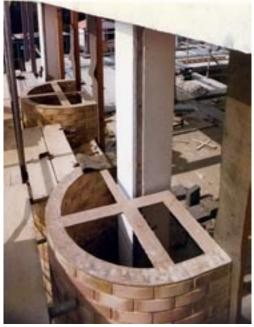
AFTER: the concrete pillar becomes merely one amongst many pieces of physical 'kit' within the ample stomach of the column of the 'Ordine Robotico'. A plywood template uses the structural frame as a trammell to guide the bricklayer upwards.
