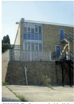
BEFORE: The Eastern end of the H.Q. Block rode out over the Warehouse forecourt on a battered retaining wall of stock bricks. Everything else was falling to pieces and not worth repairing.
