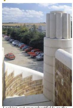
Looking-out over wheatfields on the very edge of London. The cluster of stone rods forming the Newel-cap recalls the reinforcing rods which tie the corkscrew stair together.
