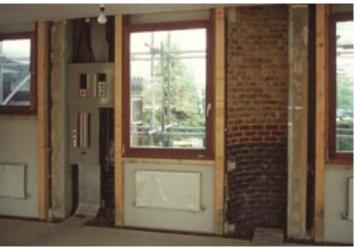
AFTER: The servicing, and the columns, are placed outside the lettable area. The brick drums were insulated internally, by foam-filled duct doors. Enough glass means small radiators. Simple and cheap.
