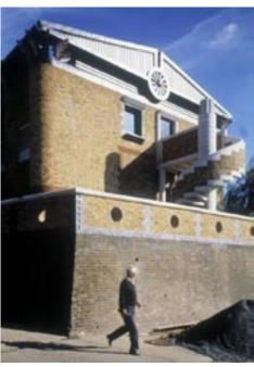
AFTER: Even though stripped to the steel frame, some old stock bricks on the 'blind' end wall were kept and patched into the new end. London stock brick was included in the the balustrade and spiral escape stair.
