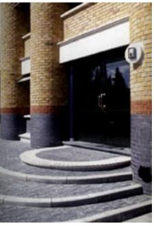
Specially pre-cast curved steps with deep anti-freezing grooves and extrasolid cantilever step-nosings.
