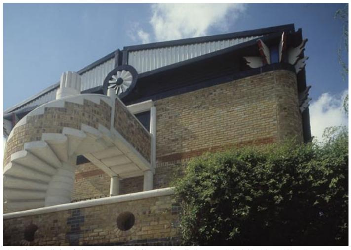
The stair descends, iconically, from the rounded beams of a raft whose rounded-off 'logs' descend from the way that the roofs of Egyptian tombs imitated unsquared timber beams. The spandrel 'ties' its bricks by compressing them with vertical s/steel rods between the precast hand rail and the precast stair treads.
