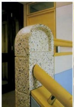
The stairs had to be remade with a steel frame. So they could carry these lovely, solid terrazzo, newels. The mixture of marble chips was precisely specified for the firm of Diespeker to cast and polish smooth.
