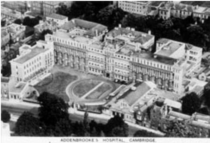
The hospital, when bought, had been continuously occupied and over-built for nearly 200 years. The facade was 19C but the buildings behind it were a labyrinth of ad-hoc 20C additions which it was aimed to demolish.
