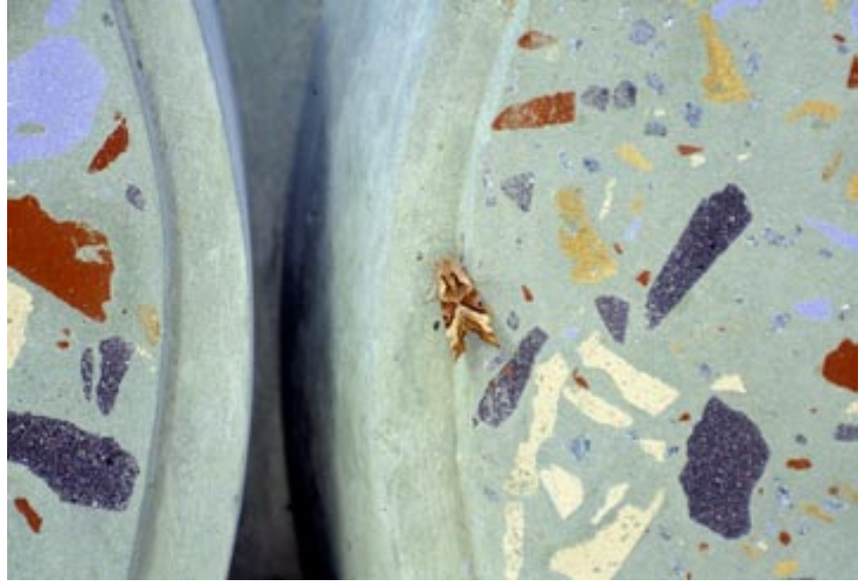
A more recent example (sporting a resident moth) of Blitzcrete' for the Millenium Verandah at Wadhurst Park. The surface of this concrete is ground back some 5 mm when still 'green' to expose the bricks. The fragments of brilliant Bayer Cobalt Blue are from bricks baked for me in the Netherlands .
