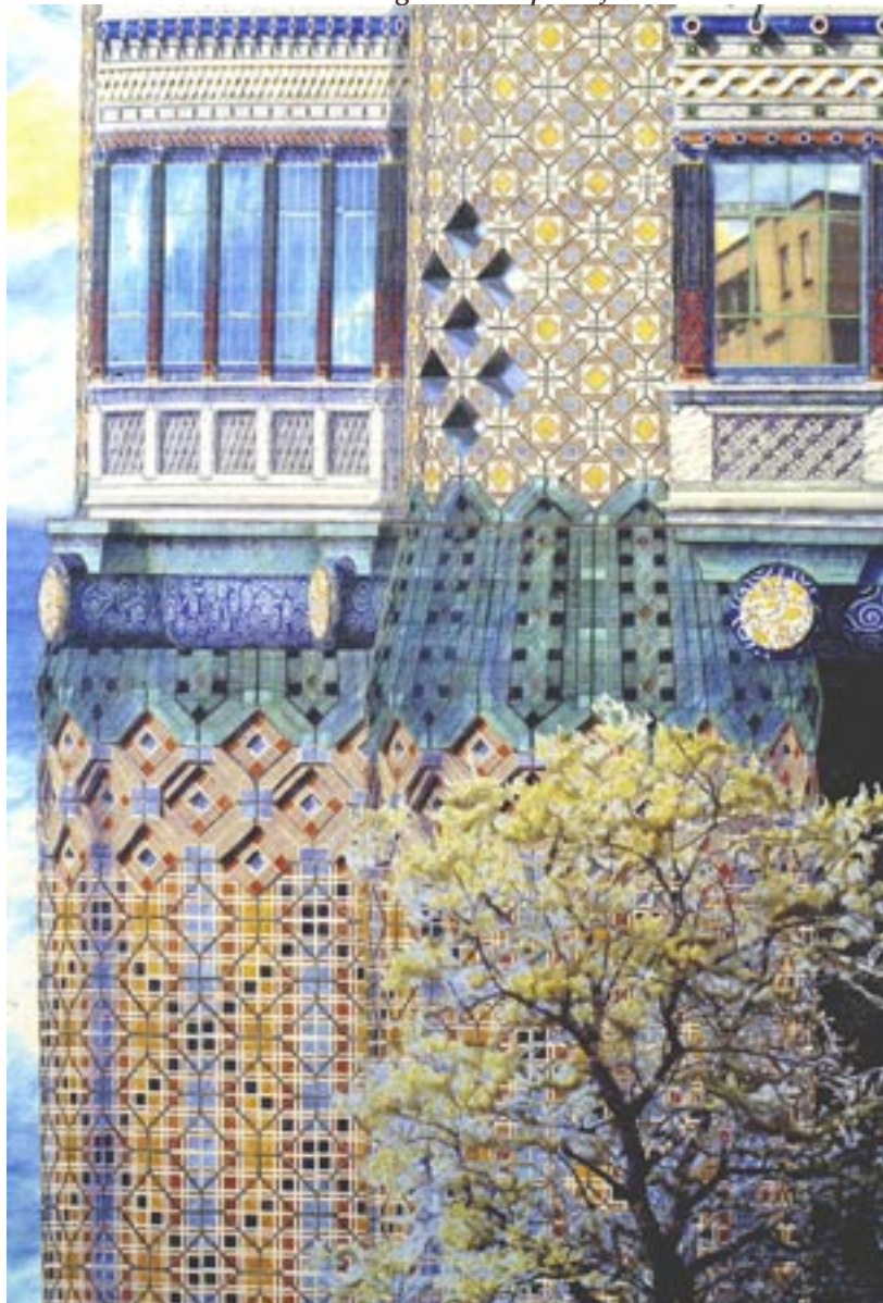
A view of the Column tiles and the window spandrels of the Blackfriars design for Rosehaugh-Stanhope. The window-spandrels were assembled from pieces of cast glass. The column changed diameter half way up. At this point the cladding was made from copper.
